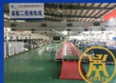
Small cabinet with assembly line
