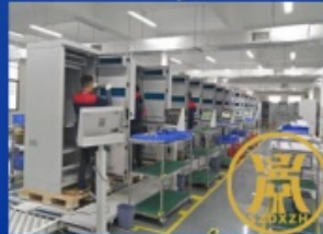
Outdoor cabinet product assembly line
