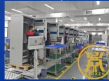
Outdoor cabinet product assembly line
